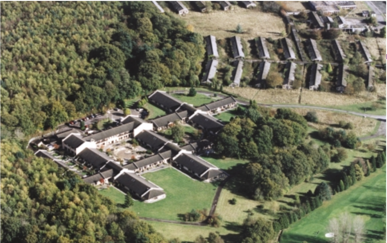
Aerial view of Ilford Park Polish Home
